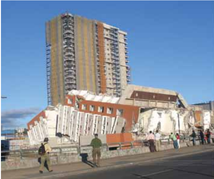
Figure 2. (Left) A toppled building in Concepcion, Chile. This failure is clearly unacceptable performance. But is the damage shown in the image on the right acceptable? It did not cause a collapse but the building is possibly unrepairable.
