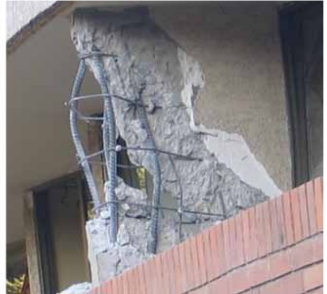
Figure 2. (Left) A toppled building in Concepcion, Chile. This failure is clearly unacceptable performance. But is the damage shown in the image on the right acceptable? It did not cause a collapse but the building is possibly unrepairable.
