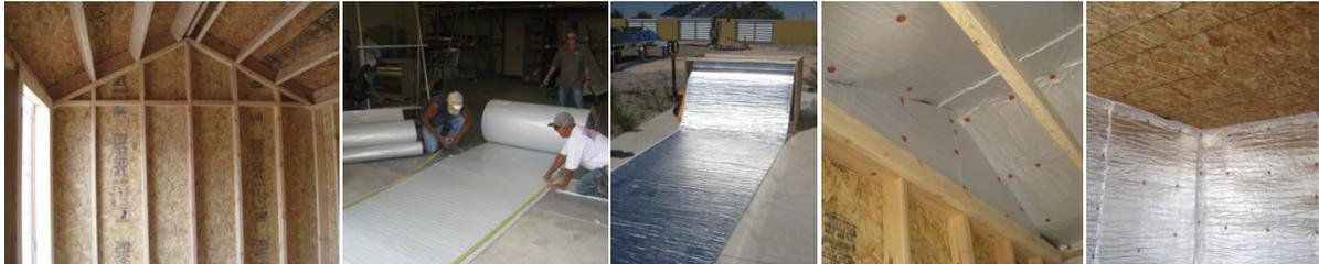
**FIGURE 2: From left to right: uninsulated hut interior prior to installation, insulation installed on roof of Hut 2, reflective insulation installed on the walls of Hut 3 with ceiling in place.**
