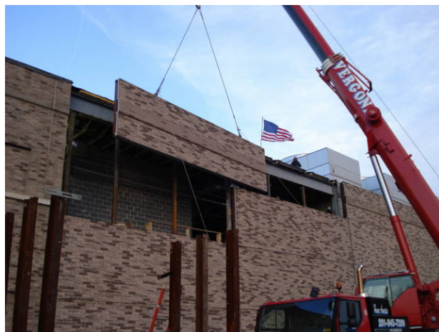
Photo 13 Steel truss with brick façade.
