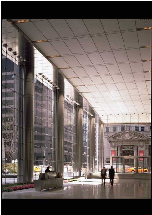
Photo 8 Cable Net wall, UBS Tower Chicago IL (Courtesy of Thornton Tomasetti)
