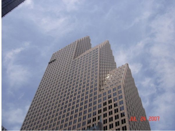
Photo 2 Curtain Wall Framing with integral granite panels Courtesy of Bank of America, Houston TX
