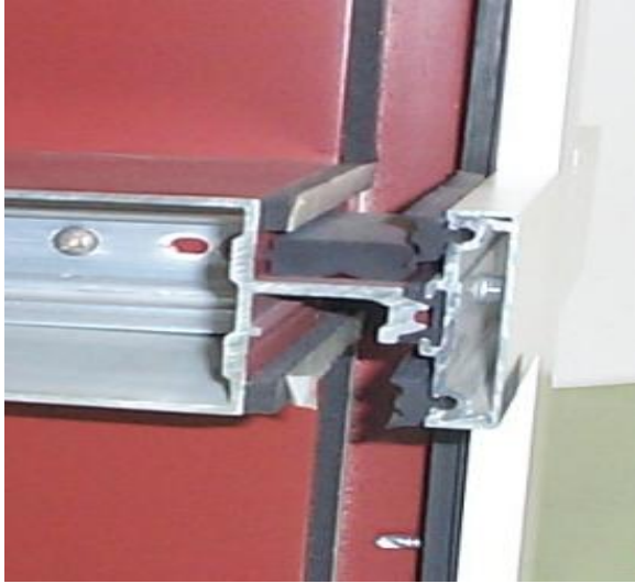
Photo 6 Typical captured aluminum horizontal framing utilizing a pressure plate system. Note the rubber gaskets in reglets and the neoprene glazing setting blocks.
