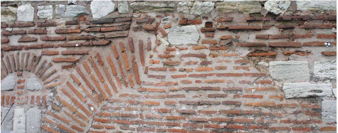
Figure 4: Exterior wall detail (Photograph by the author)
