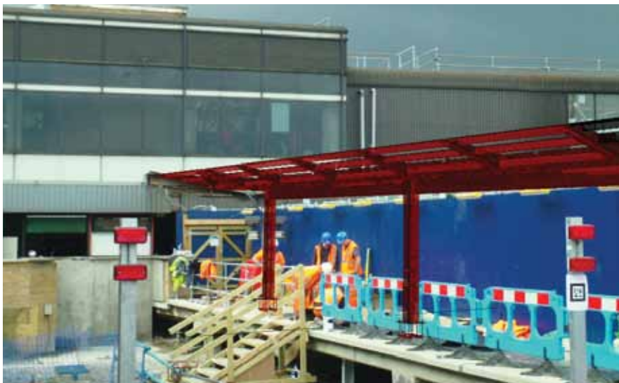
Figure 1. An AR device view of a proposed platform canopy.
