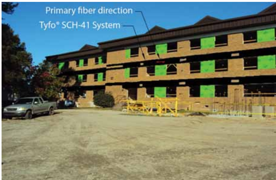
Figure 7. CFRP composite on a masonry structure for alternate load paths.
