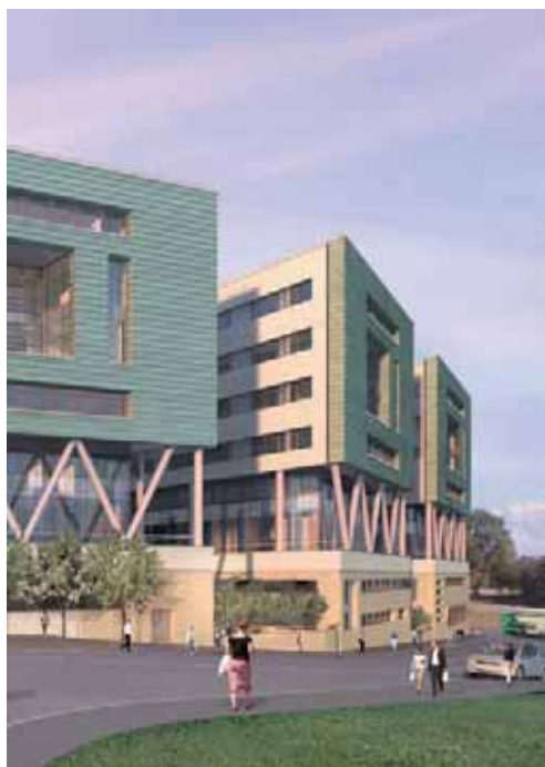
Figure 13 The New Oncology Wing is zoned vertically, with ward and outpatient areas over a podium housing radiation therapy chambers.
