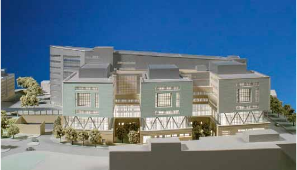
Figure 12 The finger plan surrounding landscaped courtyards enables good light and views to all patient areas.
