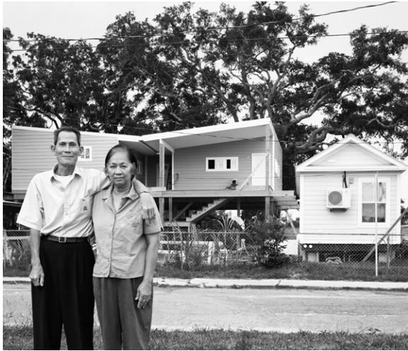
East Biloxi residents Nghia and Ban Tran with their GCCDS-designed house under construction. Image © Alan Karchmer 2008
