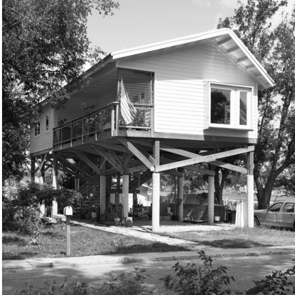
A new GCCDS East Biloxi house elevated 13' above grade. Image © Alan Karchmer 2008
