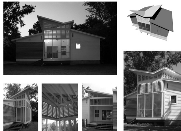
Fig. 2 DESIGNhabitat2, Greensboro, AL, 2006.
