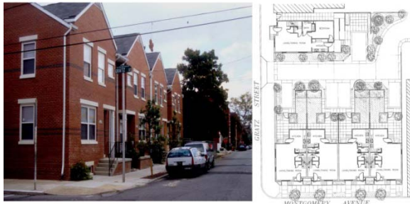
Fig. 4: Project 1800 Phase 1: Montgomery and Gratz Streets
