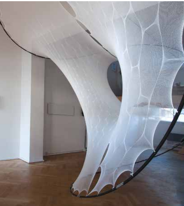
FIGURE 2. Textile hybrid prototypes developed in previous research, utilizing a CNC knitted textile as the tensile surface interconnected with bending-active
