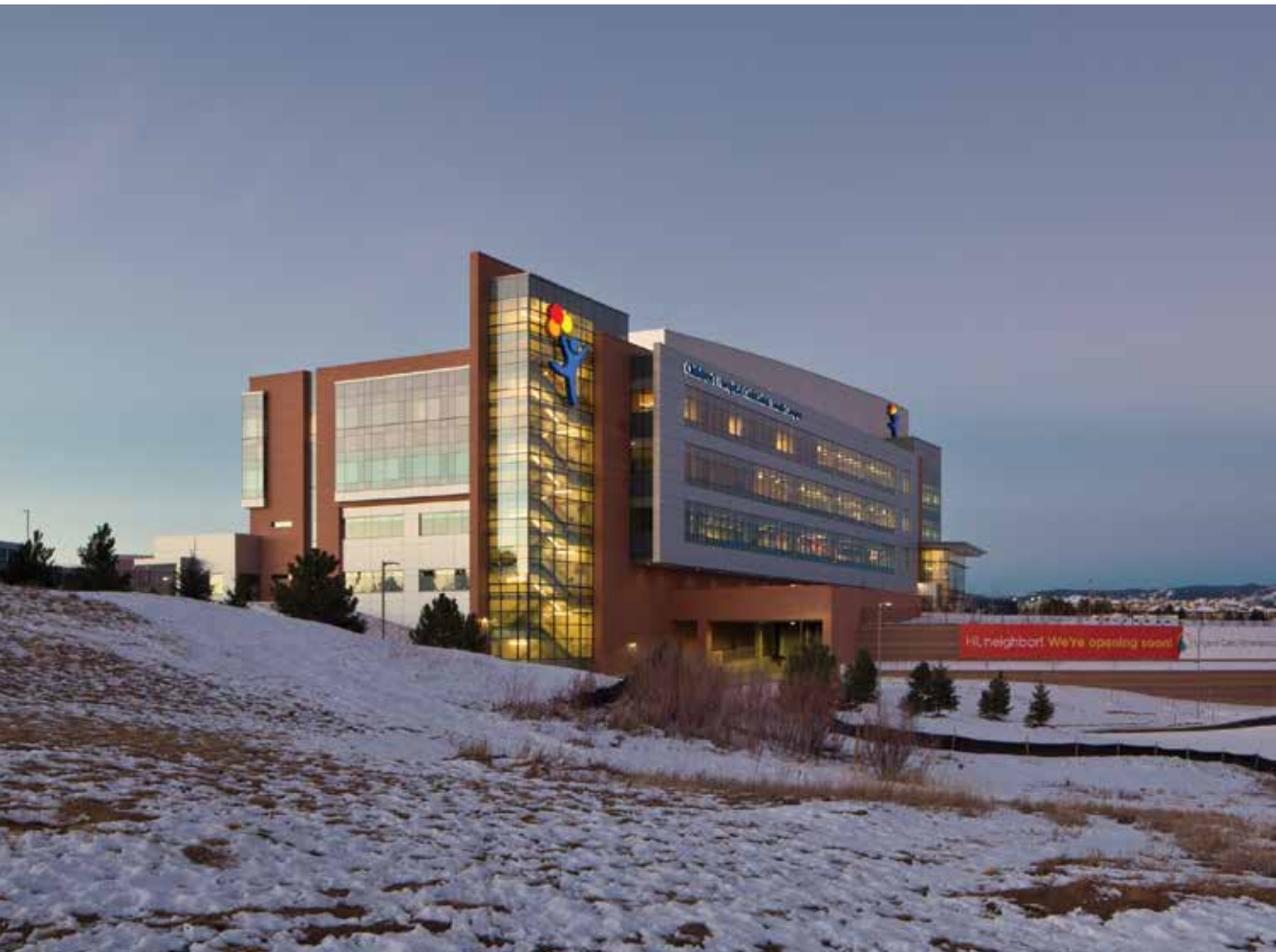
FIGURE 4. Children's Hospital Colorado-South Campus. Architect: Davis Partnership Architecture | Image credit: Brad Feinknopf
