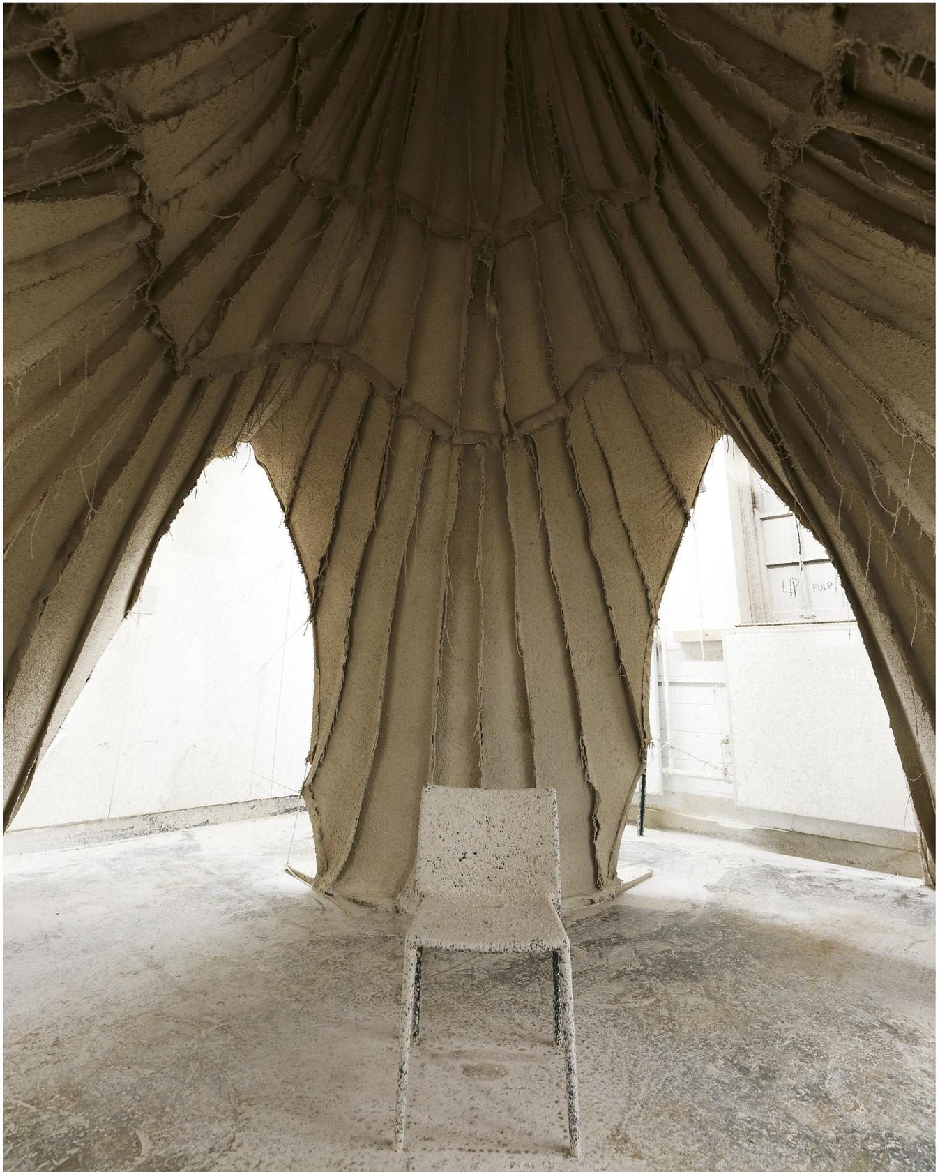
Figure 4. Interior of room scale cast paper structure made using a suspended fabric formwork. Photograph: Georg Rafailidis.
