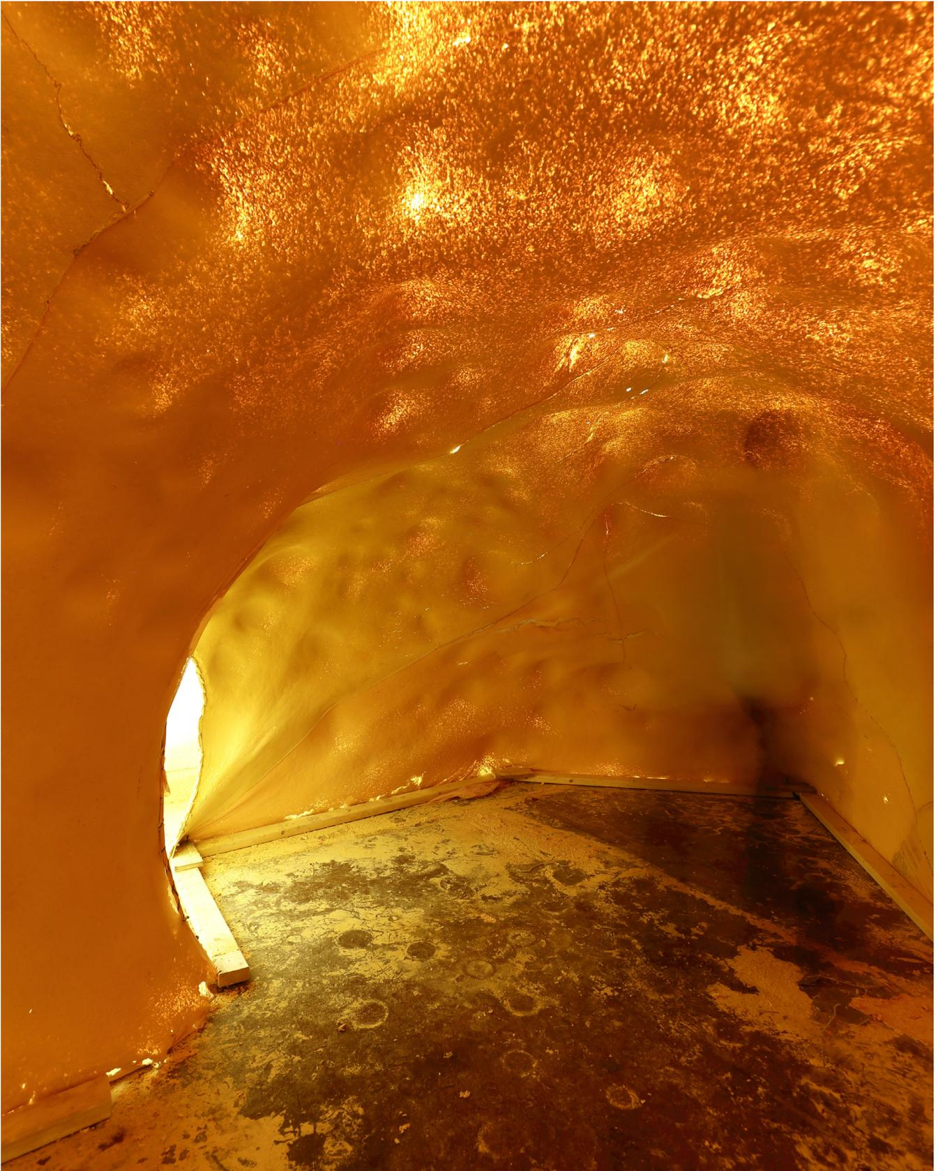
Figure 3. Interior view of room scale cast paper structure made using balloons as formwork. Photograph: Georg Rafailidis.
