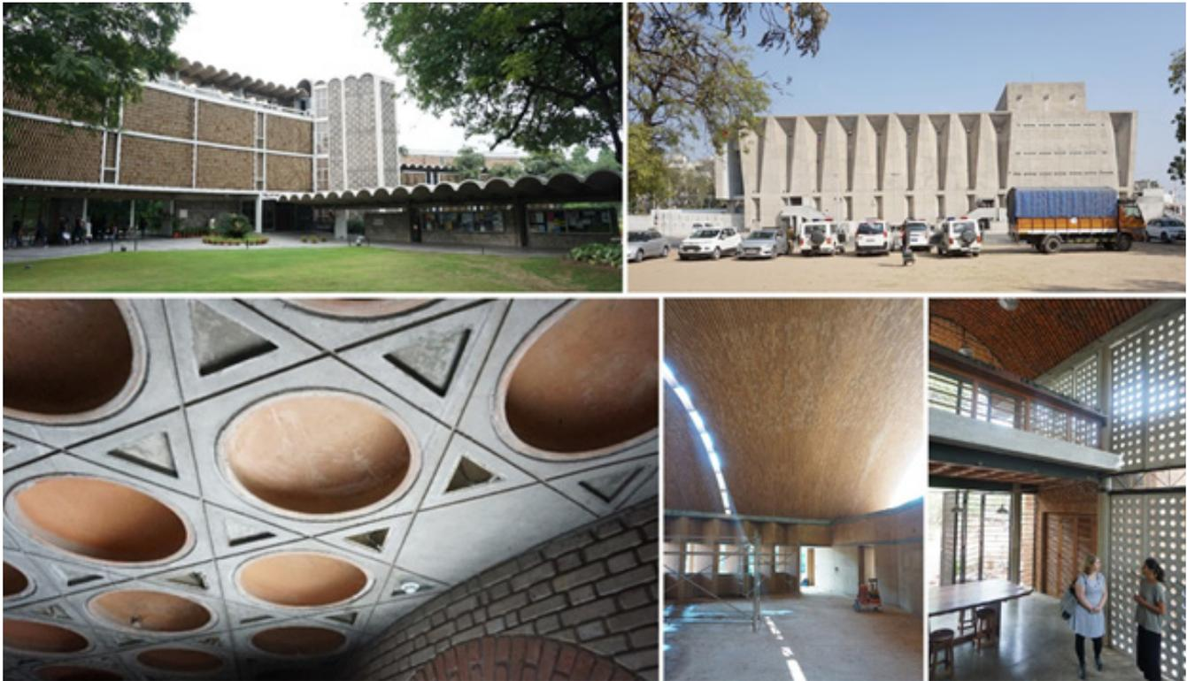
Figure 1. Clockwise from top-left a) The India International Center by J. A. Stein and Binoy Chatterjee, New Delhi, 1962 b) Tagore Memorial Hall by BV Doshi and Mahendra Raj, Ahmedabad, 1965 c) Ferrocement panels, vaulted roof, and filler slab in Wall House by Anupama Kundoo, Auroville, 2000 d) Long-spanning masonry and concrete vault at Auroville Earth Institute e) Filler slab; Development Alternatives Headquarters by Ashok B. Lall Architects, New Delhi, 2014.
