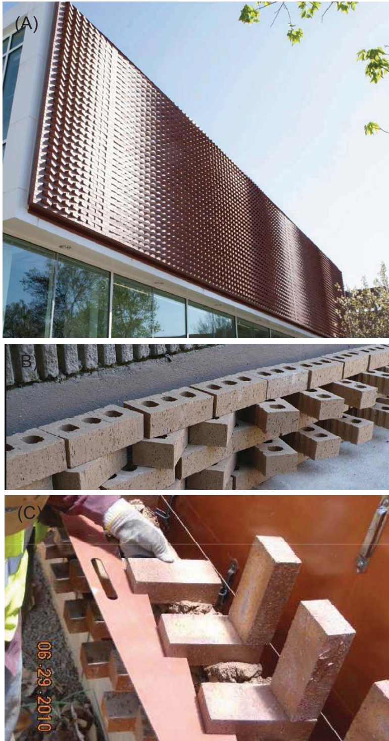
Figure 4: (A) Southern Polytechnic State University, Design Studio II, by Cooper Carry Architects, (B) conceptual strategy of brick coursework, (C) templating of rotating brick during construction (image credit: Cooper Carry Architects).
