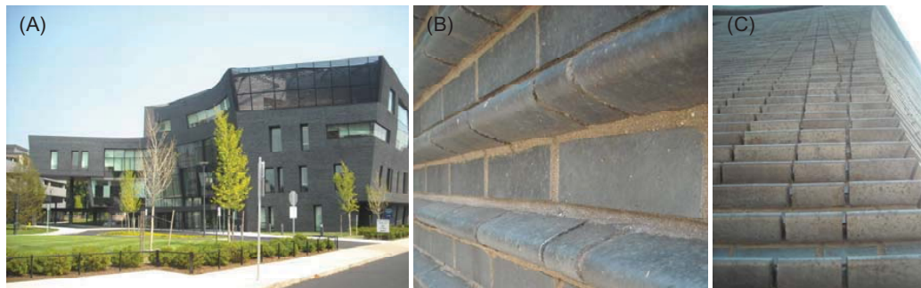
Figure 3: (A) Yale University Health Services building by Mack Scogin Merrill Elam Architects, (B) detail of bullnose brick, (C) brick coursing at non-orthogonal corner (image credit: Tristan Al-Haddad).
