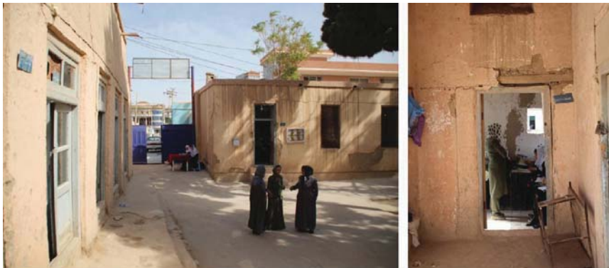
Figure 3: Existing Gohar Khaton Girls' School in Mazar-i-Sharif. Source: (Ayni Education International 2012)
