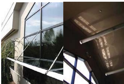
Figures 9 and 10: Left: water light shelves installed outside the windows of a Women's clinic waiting room in Eugene, OR. Right: wind-animated sunlight patterns reflected from the water surfaces of the light shelves onto the ceiling of the waiting room.
