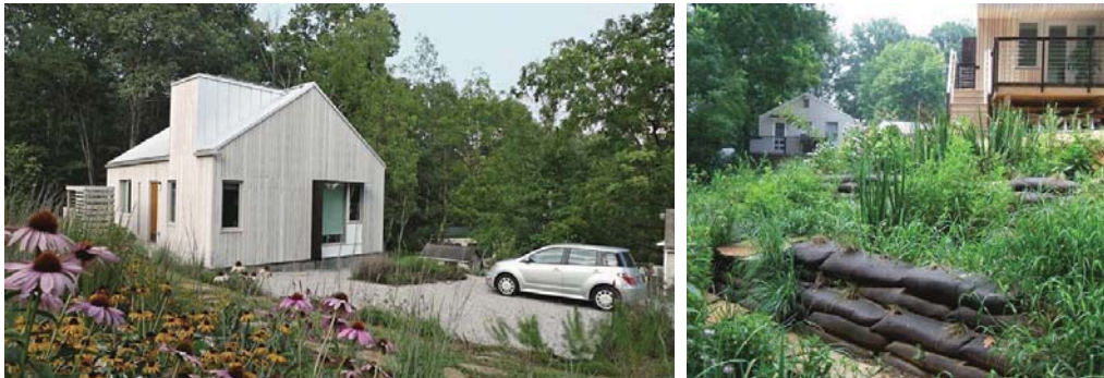
Figure 1: NNH as seen from street (left); View of greywater and rainwater infiltration bed. Bags are planted with native grasses that will eventually grow to conceal the terrace structure (right). Source: Valerie Friedmann 2012
