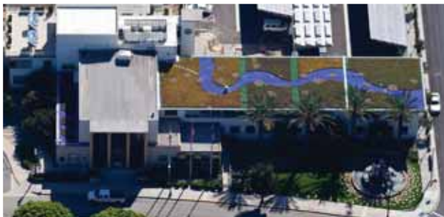
Figure 2: Green roof on Burbank Water and Power Building (California).
