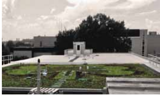
Figure 3: Green roof on Emerson Electric Company Hall (Missouri).
