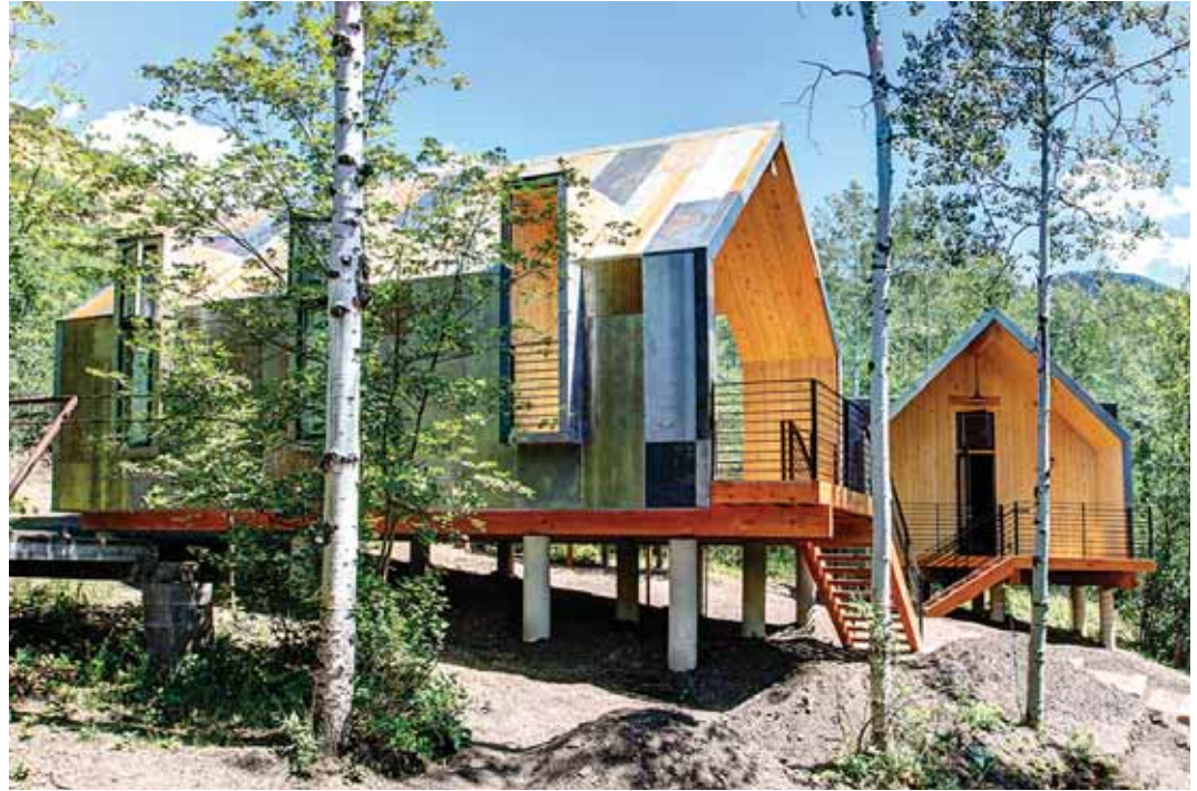
Figure 2: Completed Cabins. (Nicholas Steffens 2014)
