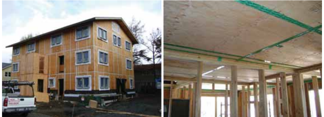
Figure 4: Taped plywood seams throughout PH.
