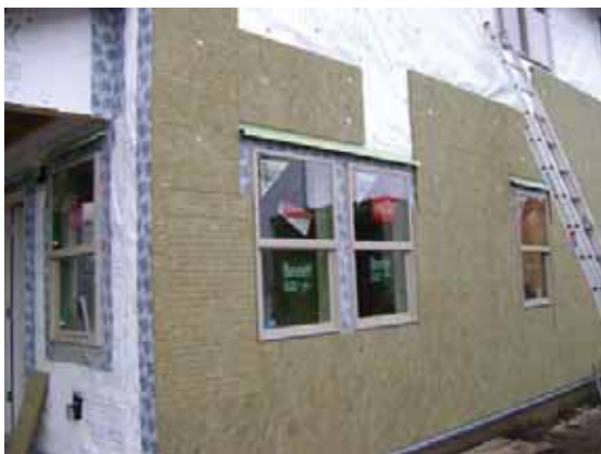
Figure 3: Continuous insulation over WRB on PHIF.
