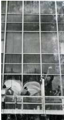
Figure 6: Lever House window washers. Source: Architectural Forum, June 1952
