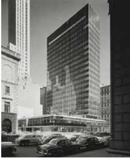
Figure 2: Lever House photograph by Ezra Stoller. (Source: www.som.com/projects/lever_house )
