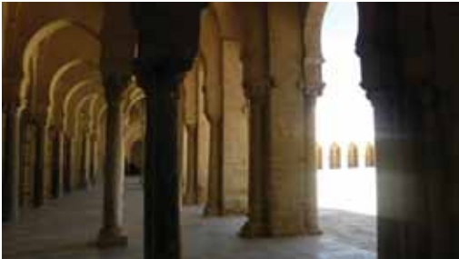
Figure 3: Interior view of the galleries. Source: (Author 2013)
