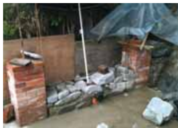
Figures 6, 7 and 8: The natural stone wall here is not a dry wall, but rather bound by mortar.
