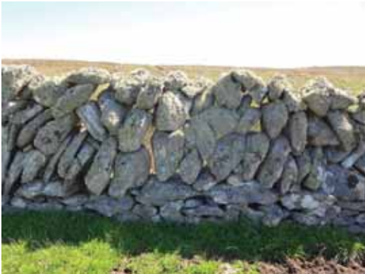
Figure 4: Galloway dyke on Fetlar, Shetland Islands, UK.
