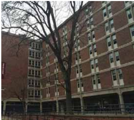
Figure 1: Grayson Hall west façade open windows.
