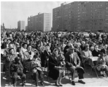
Figure 4: Photograph taken on opening day, Pruitt-Igoe project.
