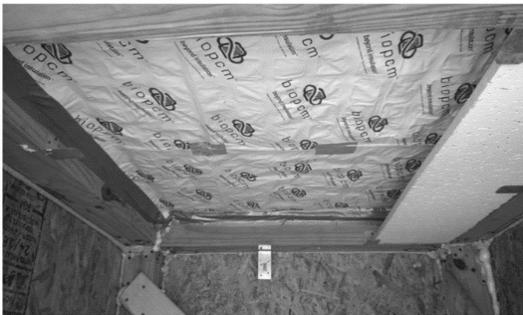
Figure 5: Installation of PCM
