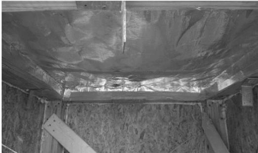
Figure 4: Installation of radiant barrier (RB)
