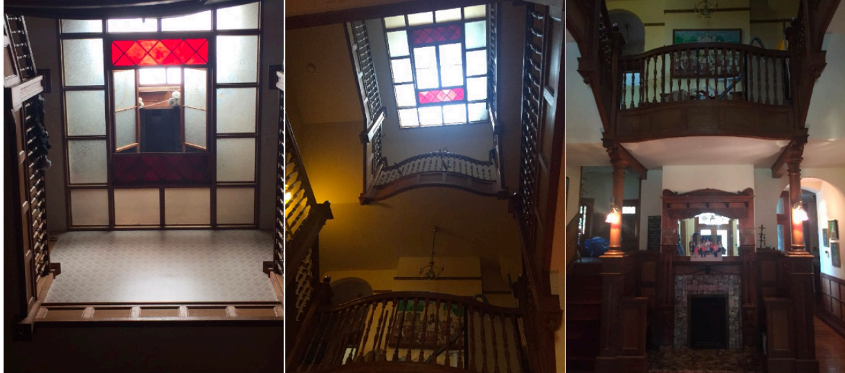
Figure 5: Images from the Kalteyer House: Ventilated shaft is surrounded by the stairwell leading to upper floors; the skylight has the dual role of illuminating the space and creating convective air flows. Source: (Author, 2016)
