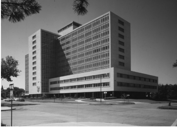
Figure 1: The Docking State Office Building soon after it was constructed. (Source: Kansas Historical Society)
