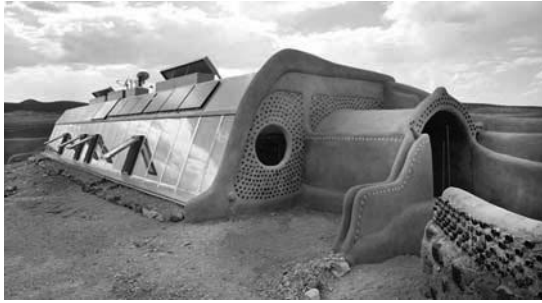
Figure 2: “South and East Side of an Earthship Passive Solar Home.” Source: (Author: Biodiesel33. Wikimedia Commons. 4 July 2011, http://en.wikipedia.org/wiki/Earthship )
