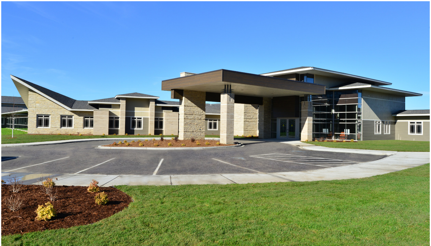
Outside view of the completed facility's entryway. Image credit: Terry Bowe
