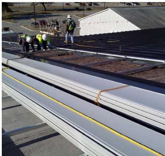
Figure 7 Gaffney Gym Solar Air Re-Roof added solar features for air inlets and outlets, solar air space zoning partitions, radiant barrier insulation, and sensors installed during construction add about $1 sqft for a roof larger than 4,000 sqft.
