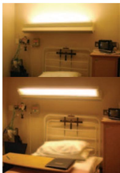
Figure 4.62 Traditional bedhead lighting is flexible for uplighting only (top) or for task lighting and medical examinations (above)
