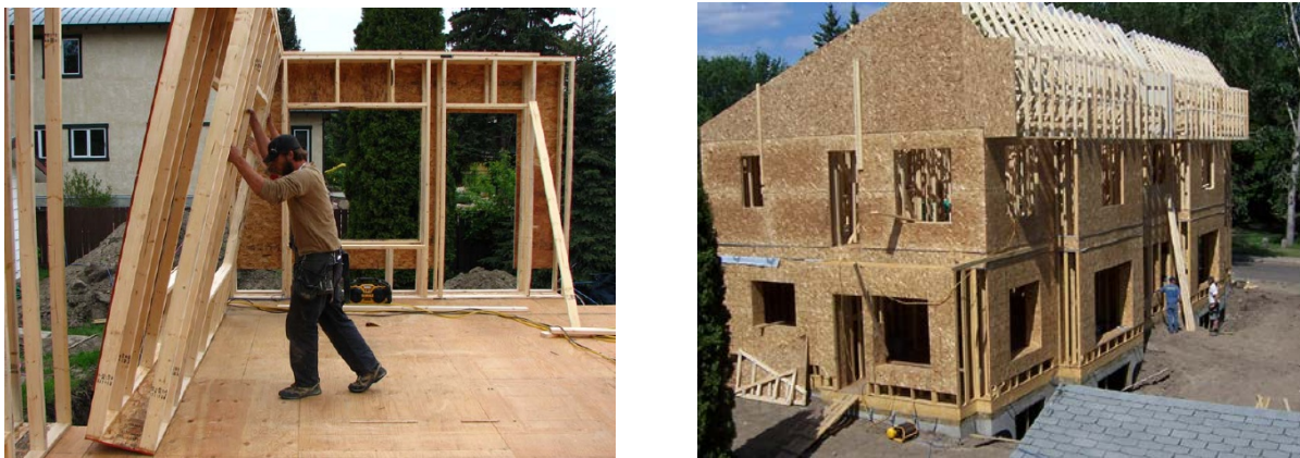
Figure 2. Double wall construction (Riverdale Net Zero Project, 2007)
