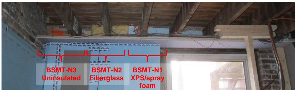
Figure 3: Comparison of insulation strategies for joist ends BSMT-N-1/2/3, pre-drywall
