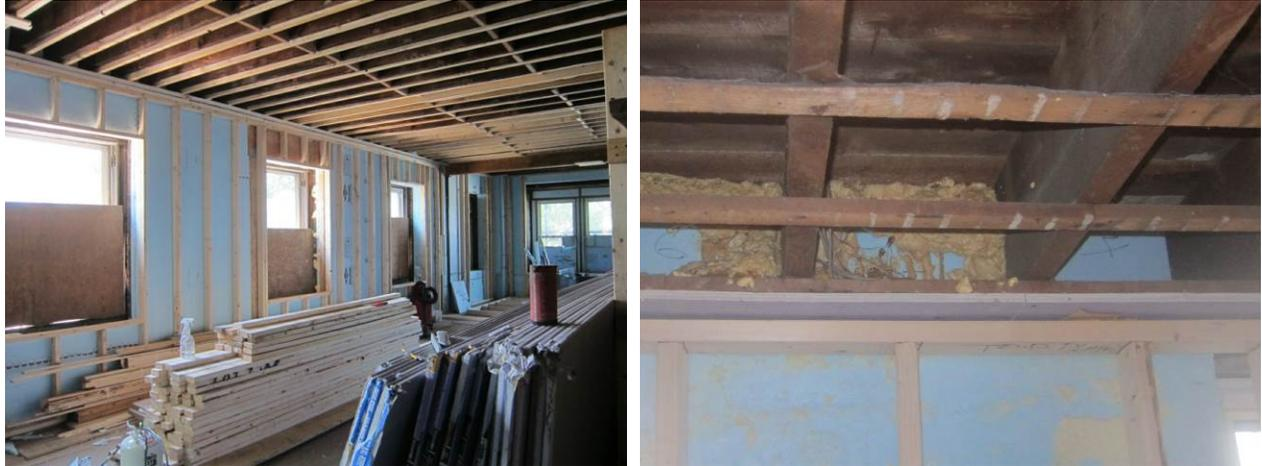
Figure 2: Framing installed inboard of insulation (right); insulation and air seal at joists (right)
