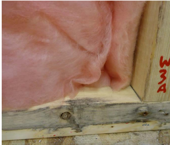
FIGURE 10: West Wall 3A Bottom Plate. Note: Staining is visible on the interior surface of the bottom plate where water has drained down the poly and become trapped at the bottom between the taped edge of the poly and the wood. This was the worst observed staining of all poly walls. Some staining is also evident on the side of the vertical stud at the interior edge.
