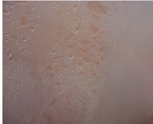
FIGURE 11: West Wall 3B Poly. Note: There was sufficient condensation on the poly to accumulate into large, easily visible drops. When there is sufficient accumulation, it will drain to the bottom plate, and wet the insulation in the cavity. In some of the poly walls, there was only a little condensation, which had not yet formed large droplets.
