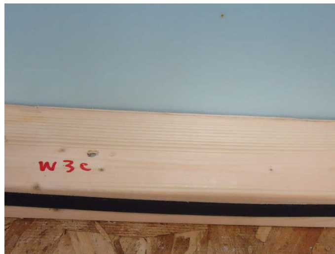
FIGURE 12: West Wall 3C Bottom Plate and XPS. Note: There is no staining on the top or inside edge of the bottom plate, or on the surface of the XPS. There is no corrosion of the fastener in the bottom plate.
