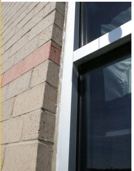
Design should account for consequences of aging/failing of seals and gaskets
