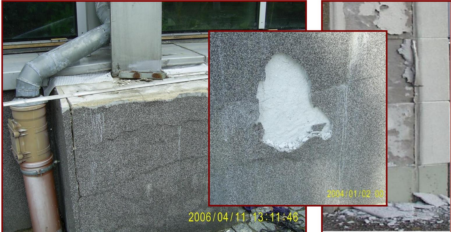
Frost degradation of the plaster in the climatic conditions of Poland,
