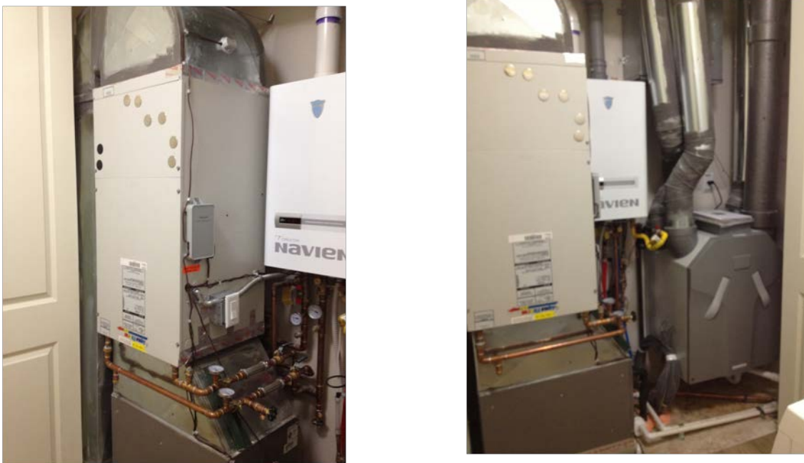
FIGURE 4: Mechanical closet with the air handler and water heater (left) and the ERV (right)
