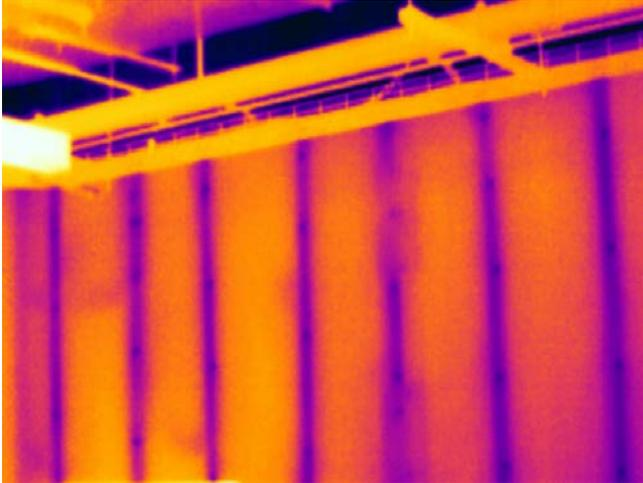
**Figure 12 : Infrared image showing studs attached directly to exterior masonry wall**
