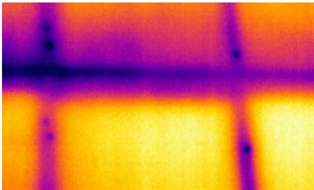
**Figure 6 : Thermal Image of Z-girt Support for a Rainscreen**
