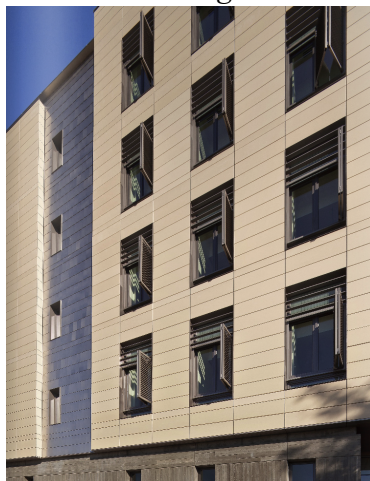
Li Ka Shing, UC Berkeley campus Aluminum louvers above window Aluminum louvers in shutters (shd 8)
