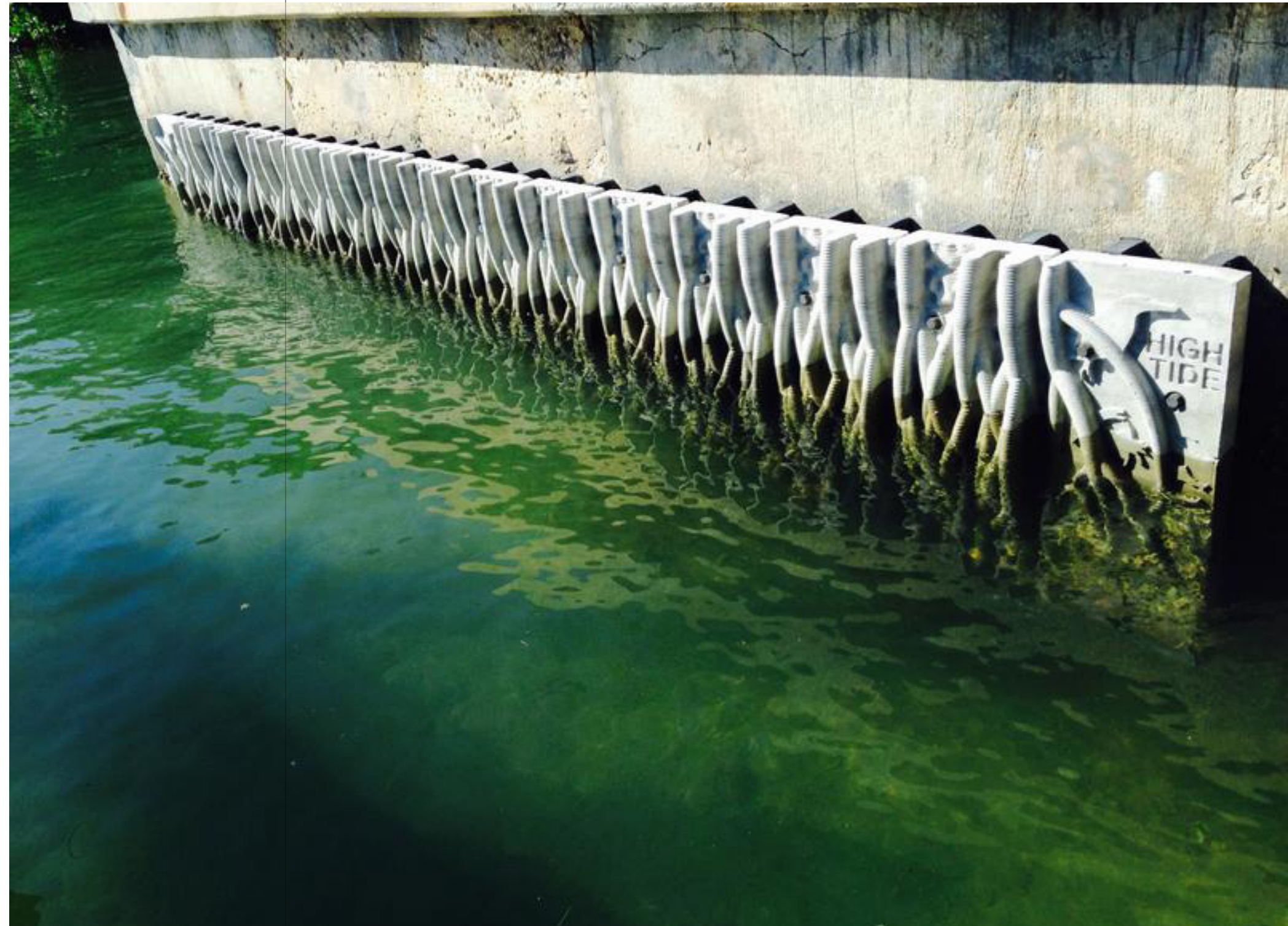
Figure 1. Prototype panels installed on Manasota Key in Englewood, FL in 2016. Image credit: WGPU Radio, Fort Myers
