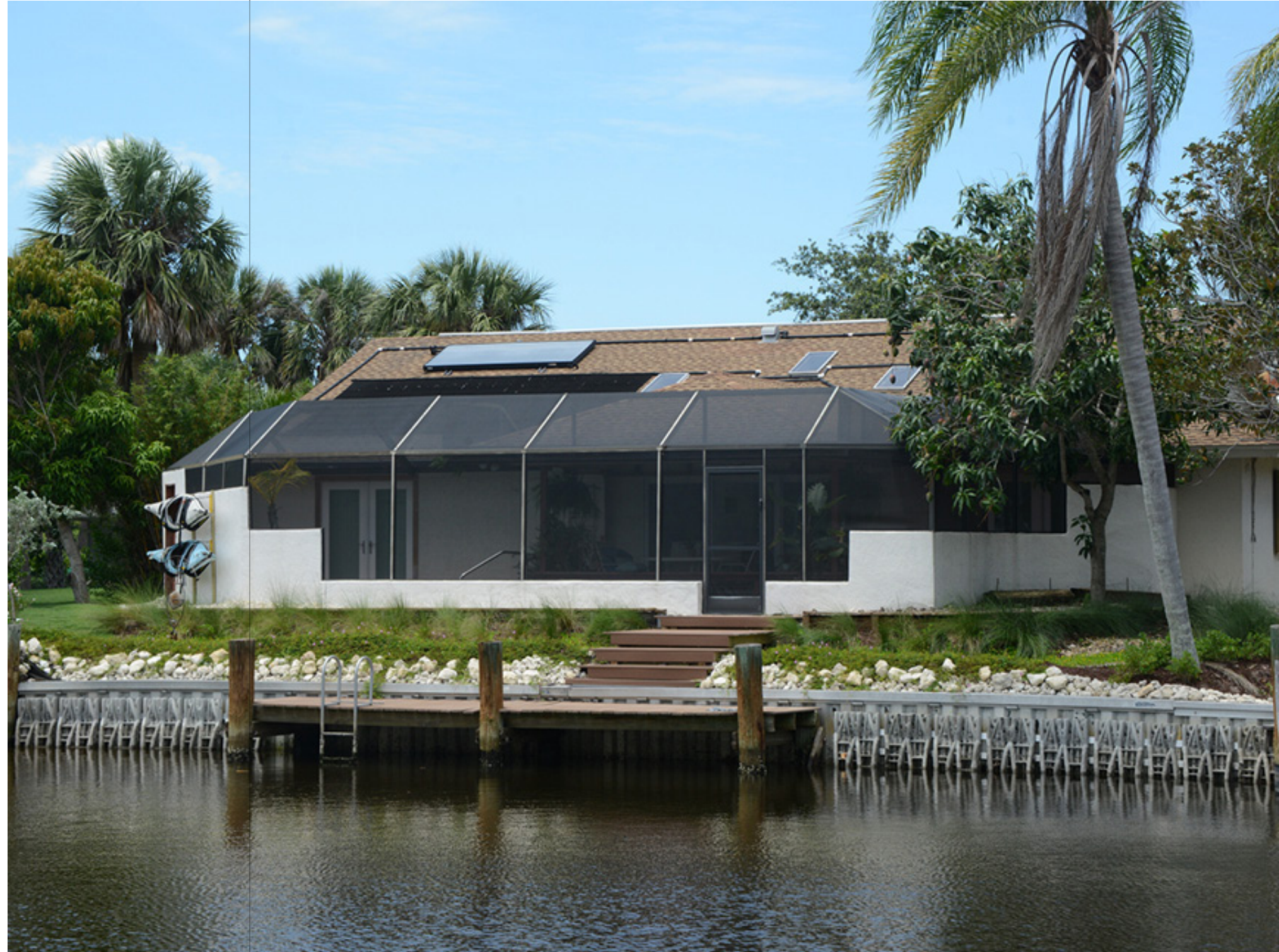
Figure 22. Fort Pierce seawall installation. Landscape architect Meg Whitmer designed native plantings over a limestone berm adjacent to the seawall. Image credit: Dr. Edith Widder, ORCA
