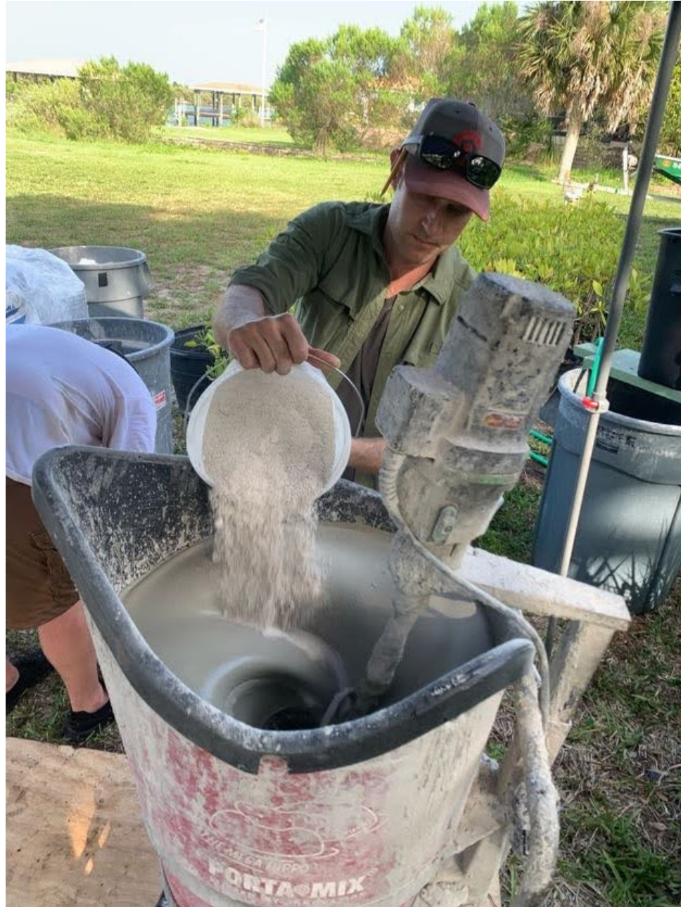
Figure 23. Panels for the Fort Pierce installation were 24"x36" and cast with a silicone rubber mold. Roots extended approximately 12" outward from the seawall face. Oyster flour (above left) was added to the concrete mix to be marine-friendly.
