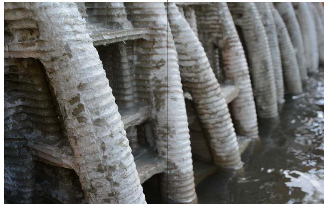
Figure 24. Other than a few barnacles (left), the corrugated aluminum seawall had virtually no biological growth prior to installation. The panels were installed summer of 2018 (center) and periodically monitored. After a slow start, the recruitment of oysters and barnacles accelerated to completely cover the panels (right).
