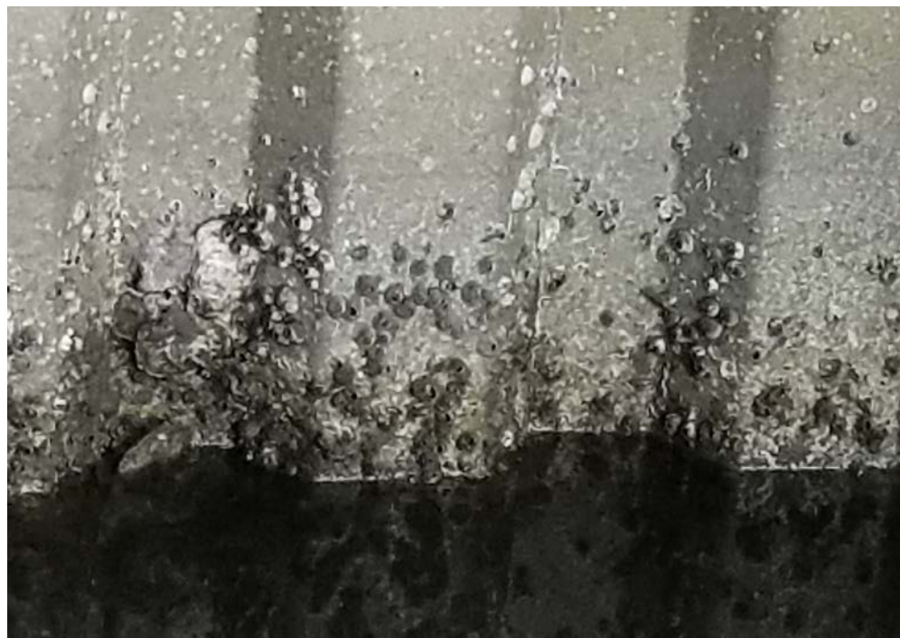
Figure 24. Other than a few barnacles (left), the corrugated aluminum seawall had virtually no biological growth prior to installation. The panels were installed summer of 2018 (center) and periodically monitored. After a slow start, the recruitment of oysters and barnacles accelerated to completely cover the panels (right).
