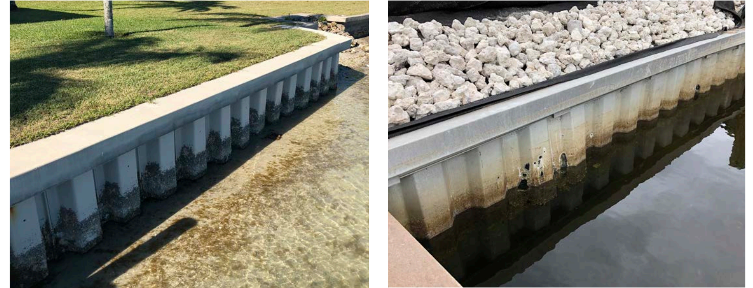
Figure 13. Over the past few decades, vinyl and metal sheetpile seawalls have gained traction. Whereas concrete seawalls host some oyster growth, these walls have little to no biological recruitment and are worsening the impact of seawalls on the marine environment.
