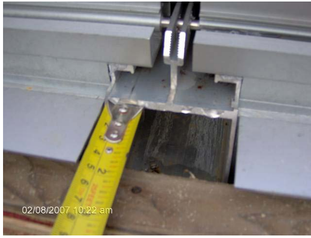
PHOTOGRAPH 12: Exterior view of a raised leg skylight with overlapped drainage gutters.
