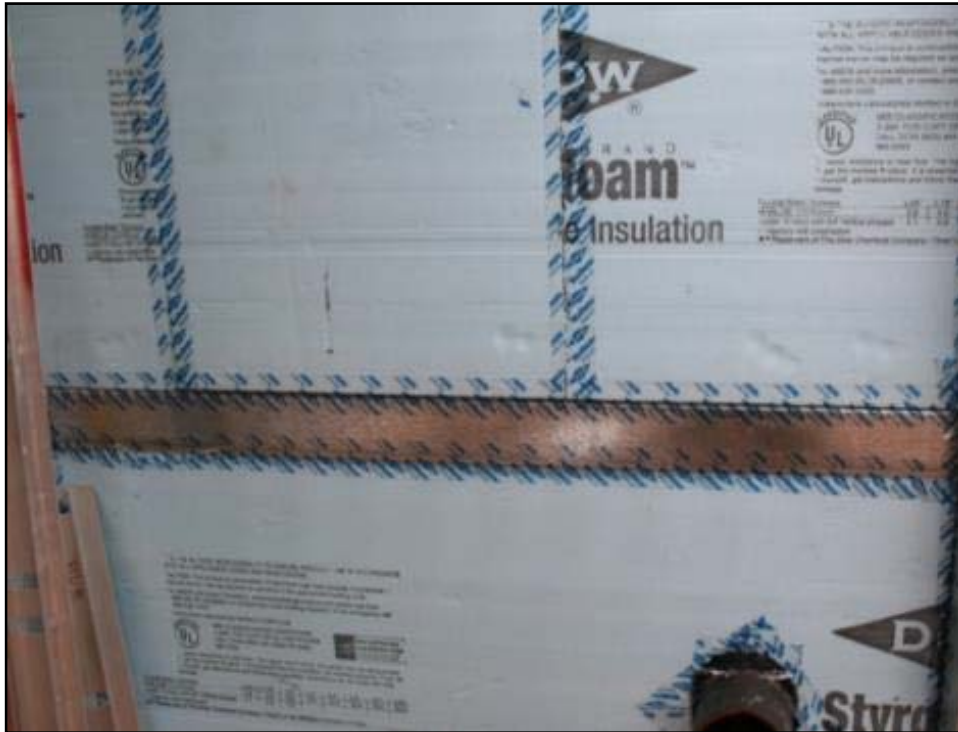
Taped Insulation Joints
