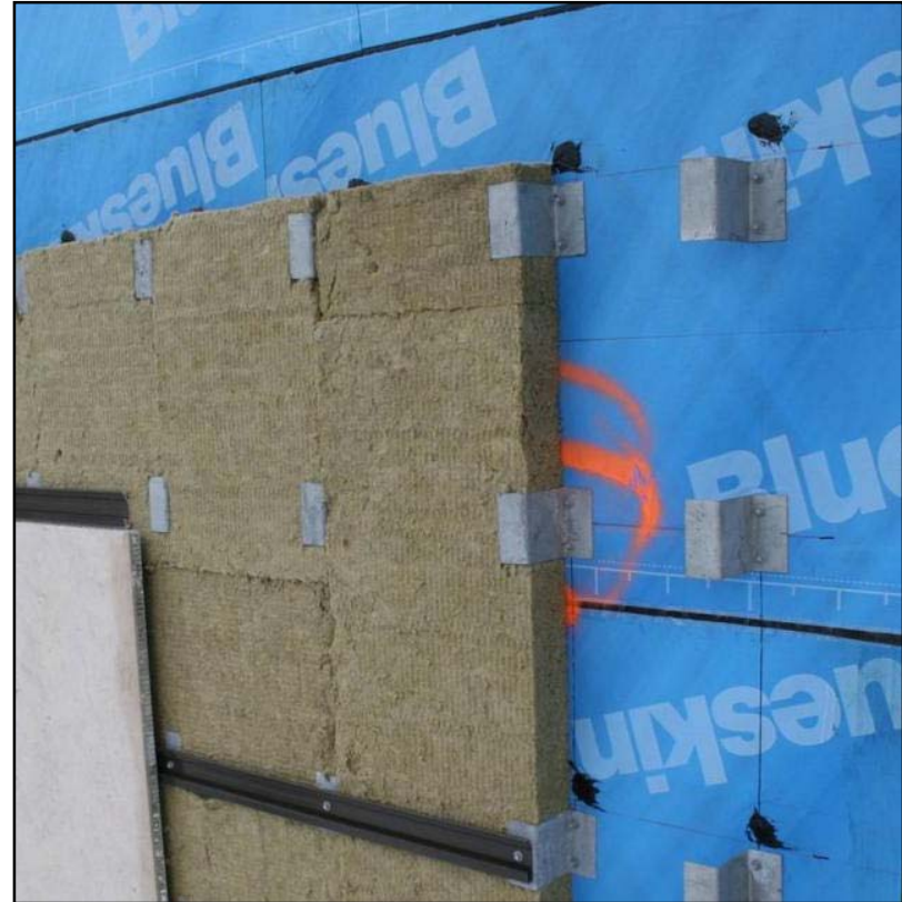
Tight Insulation Joints
