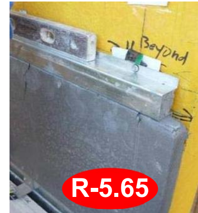
High R - Extruded Polystyrene (XPS) 1.75" = R-10 // 2.125" = R-12
