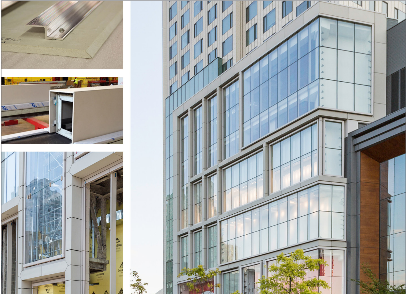
FIGURE 11 A\UHPC cladding a Unitized BVDC integrated with glazing system. This example from a multi-use retail and residential complex in New York responds to the architects' desire for more expression of architectural depth on the facade of the building than the layers of the wall actually require.
