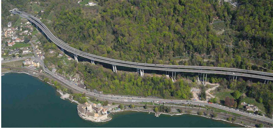
FIGURE 2 Chillon Viaduct, Geneva Switzerland, road surface topping with UHPC
