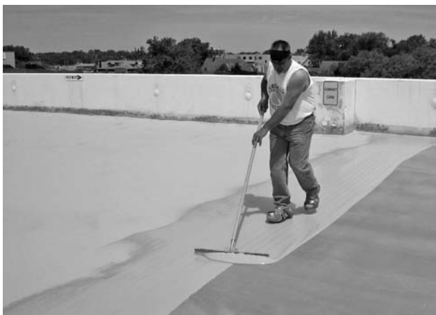
▲ Installation of a traffic-bearing membrane involves multiple steps, including application of a liquid-applied coating ( left ) and integration of a textured wearing surface ( right ). The resultant membrane protects against corrosion, but requires maintenance and periodic reapplication.
