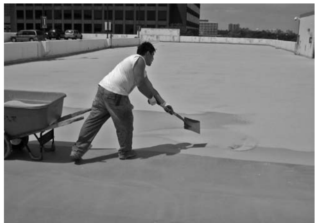
▲ Installation of a traffic-bearing membrane involves multiple steps, including application of a liquid-applied coating ( left ) and integration of a textured wearing surface ( right ). The resultant membrane protects against corrosion, but requires maintenance and periodic reapplication.
