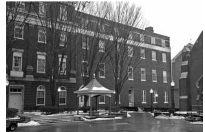
▲ Georgetown University, Former Jesuit Residence (Ryan and Mulledy Halls) in Washington, District of Columbia. Exterior Restoration Consultation.
