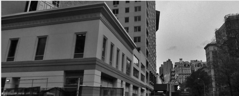
▲ Overcladding of an existing brick masonry building with exterior insulation and finish system (EIFS).
