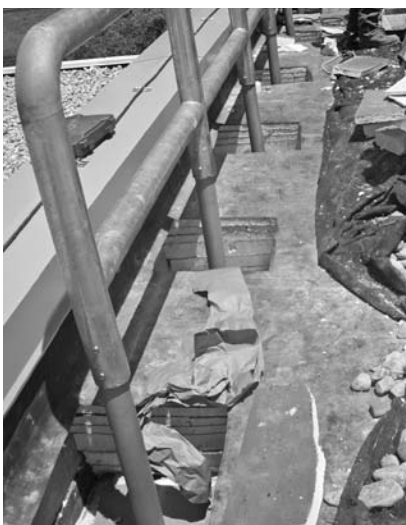
▲ Considerations for railing installation at this roof include thermal bridging and achieving correct railing height due to added insulation.
