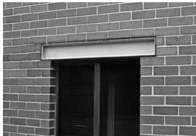
▲ This steel lintel acts as a thermal bridge, conducting heat through the building exterior.
