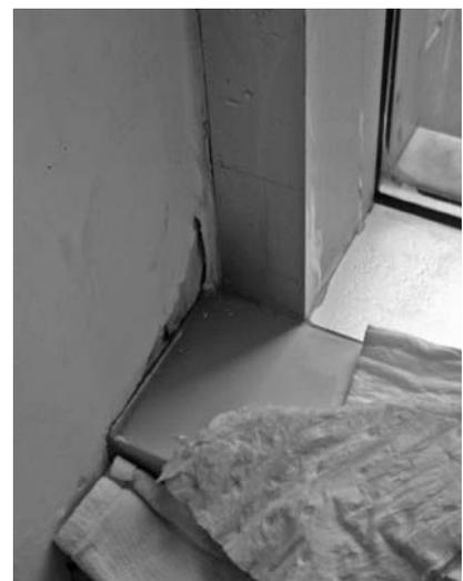
▲ New high-performance windows installed adjacent to conductive wall assemblies can still lead to condensation and moisture damage.
