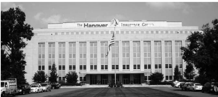
▲ The Hanover Insurance Group Headquarters in Worcester, Massachusetts. Window and Curtain Wall Replacement Design Study.
