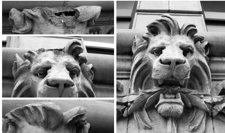
▲ Restoration of spalled terra cotta decorative element.
