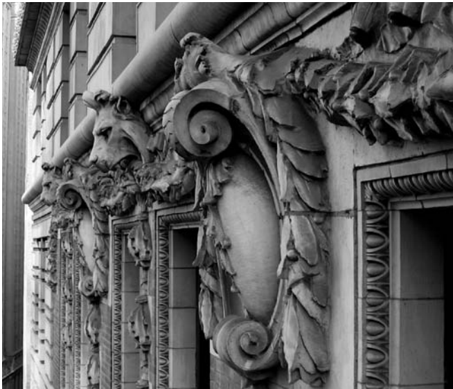
▲ Often finished in imitation of stone, terra cotta can be difficult to recognize and may be mistaken for cast stone, concrete, stone, or brick.
