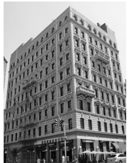
▲ Hotel Wales in New York, New York. Landmark Terra Cotta Repair and Replacement.
