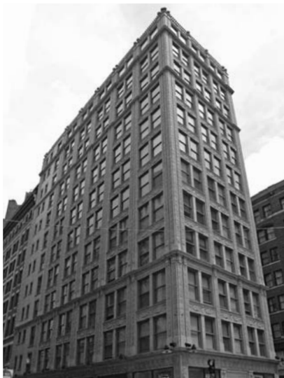
▲ Chauncy House in Boston, Massachusetts. Facade Investigation & Terra Cotta Repair Design.
