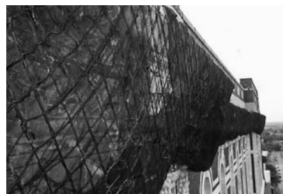
▲ Until permanent repairs are made, netting may be used to secure unstable terra cotta.
