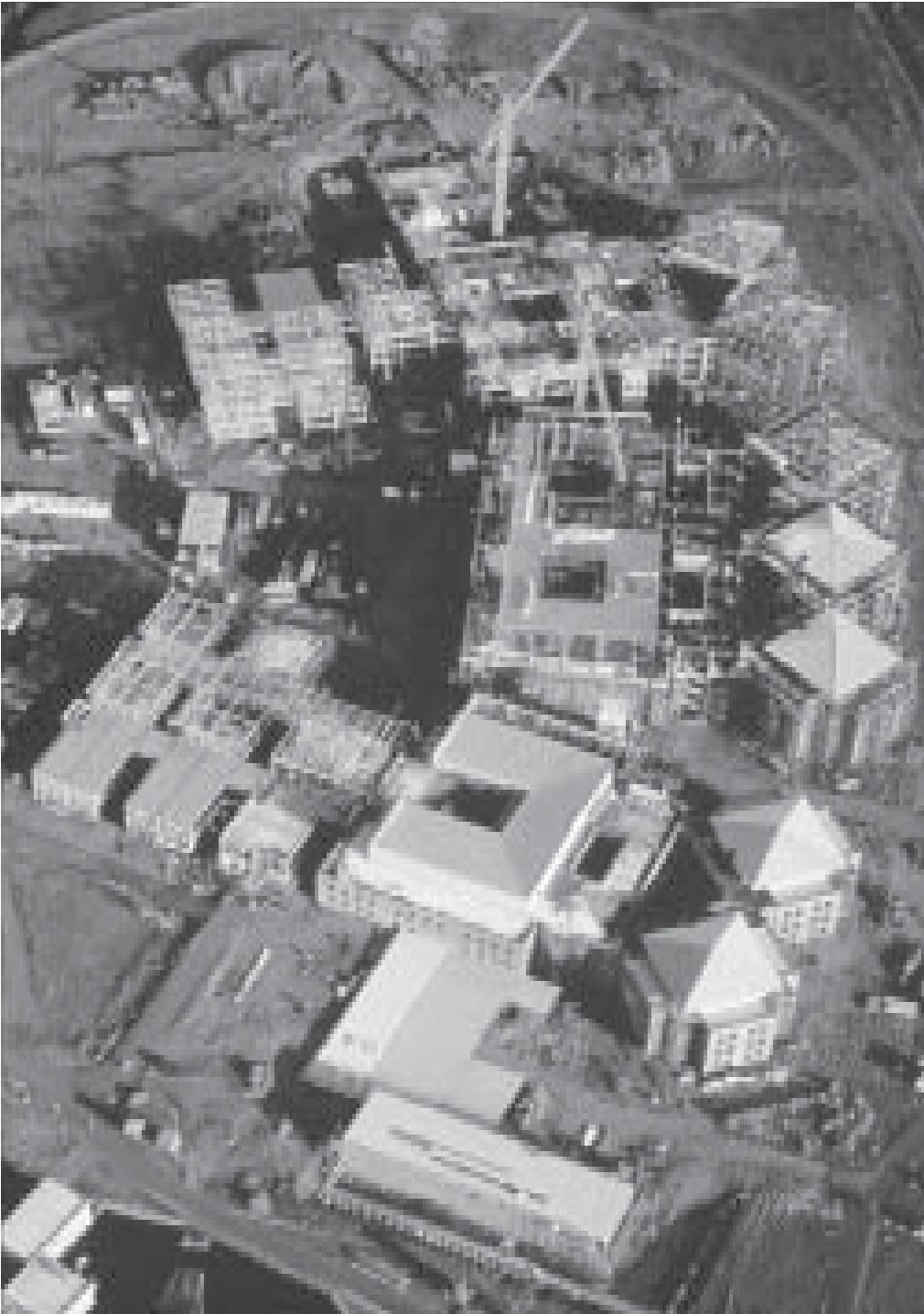
The Norfolk & Norwich PFI Hospital under construction.
