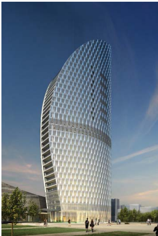
Figure 18: Inclusion of aluminum panels in building facade.
