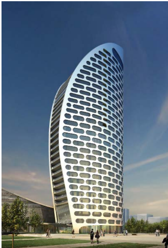
Figure 8: Flat 2D façade; Oval curtain wall option.
