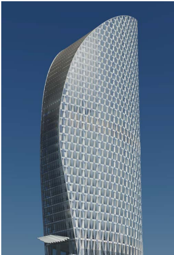
Figure 20: Flattened 2D curtain wall version of the faceted diamond option.
